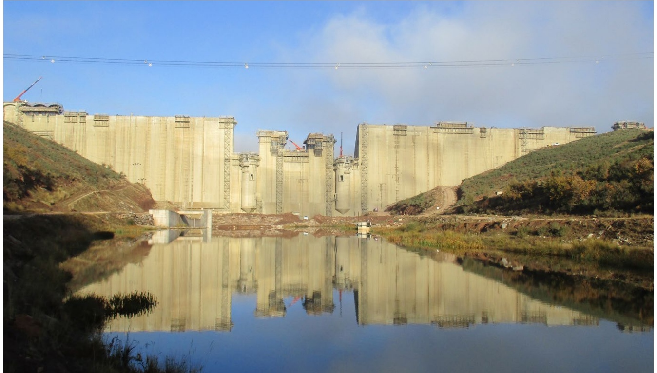
Castrovido Dam, Burgos (Spain)
