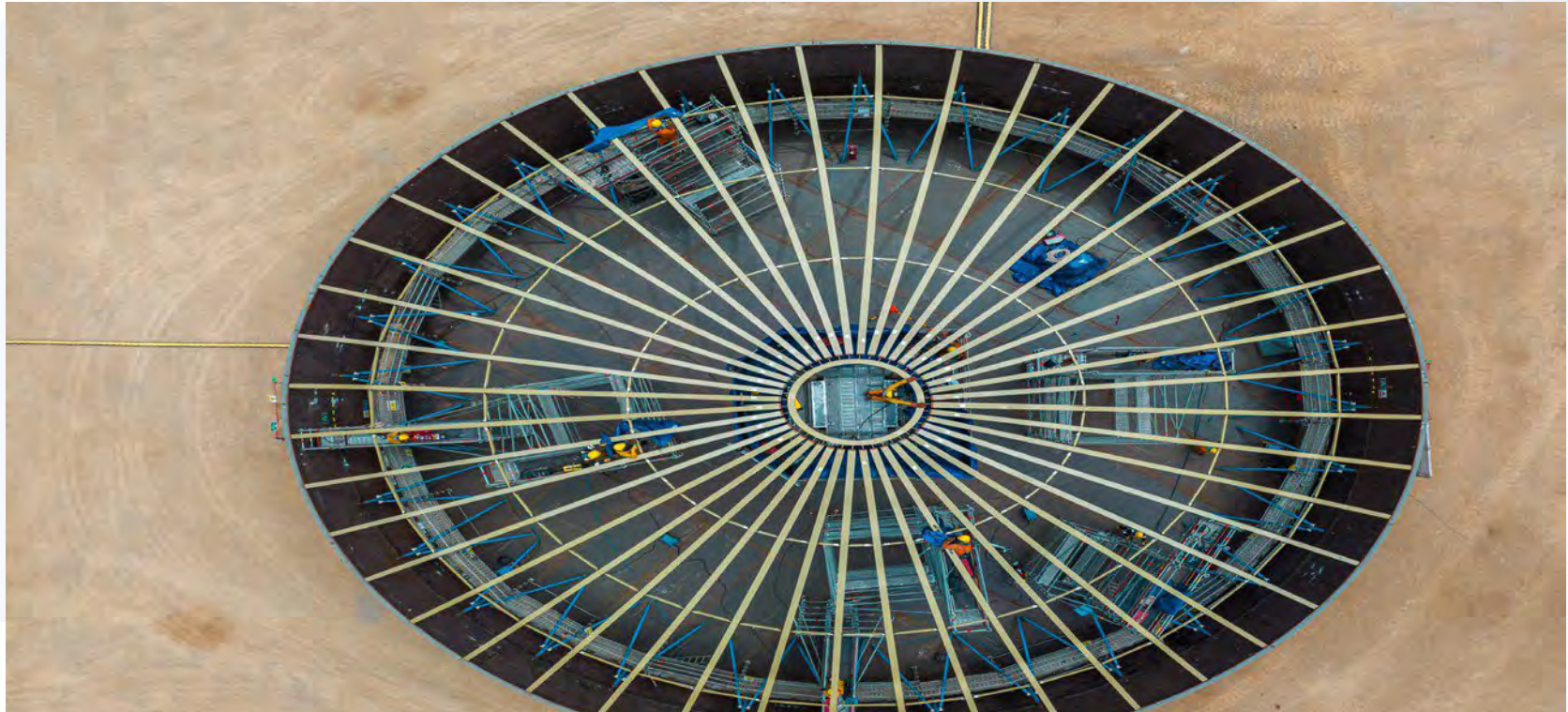
Fuel storage tanks A. International Lima/ Peru
